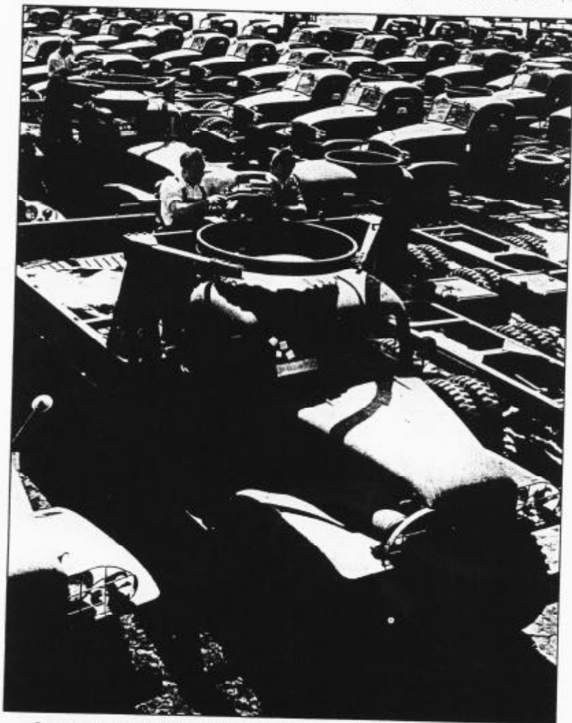
Somewhere in the Mediterranean theater, a wad of long wheelbase cargo trucks are being assembled and fitted for M-32 ring mounts. Both steel and wood bodied trucks are in this view.
