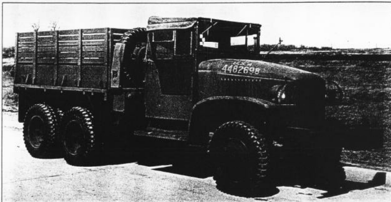
Right-front 3/4 Portrait view of a true classic. Points of interest to the collector in this May 1943 view: the last use of the large 4" numbers, the early style (1942/43) canvas with the floppy top and the large/small side curtain windows. Note also, no gas can holders on the running boards, but the large gas fillers have appeared. And, of course, the standard wartime wooden cargo body. Less than 10% of the CCKW's were the short wheelbase version. April 13, 1943.
